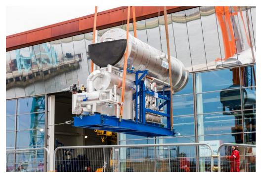
Figure 2 – A river source heat pump (2,650 kW heating capacity) delivered to Queens Quay, Clydebank
