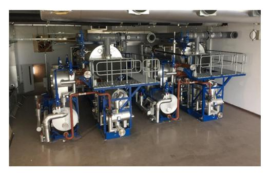
Figure 3 – The two heat pump systems (each 2,650 kW heating capacity) in the energy centre
