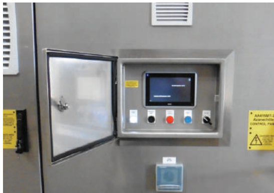
Stainless Steel Control Panel For extended life in outdoor operation.
