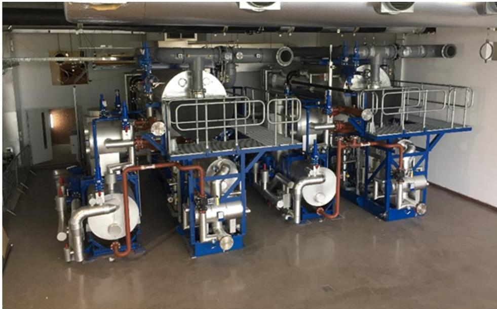
**Figure 3 – The two heat pump systems (each 2,650 kW heating capacity) in the energy centre**
